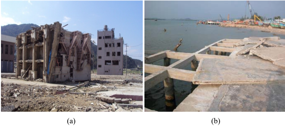
Figure 2.17 Damage to reinforced concrete structures caused by tsunamis: a) overturning of apartment building, Onagawa, Japan 2011; and b) uplift of slabs in Khao Lak, Thailand, 2004 (Saatcioglu et al., 2009)
