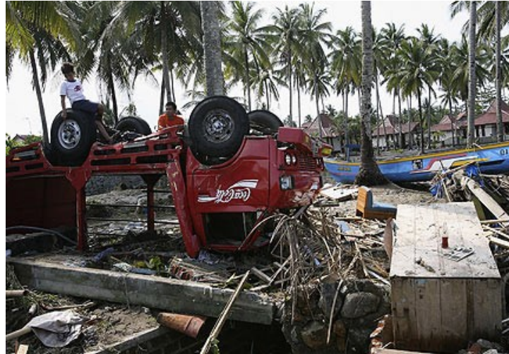
Figure 2.3 Damage due to tsunami in Papua New Guinea (July 1998) (PMEL, 1998)
