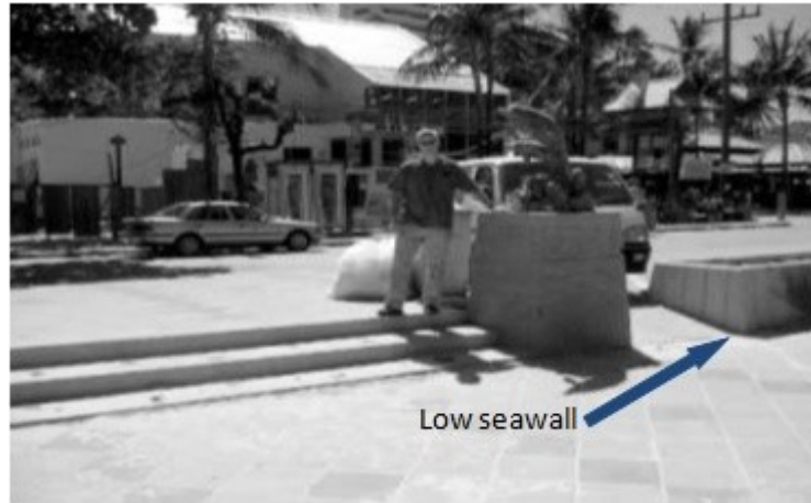
Figure 2.28 Pedestrian opening in the Patong Beach seawall (RCDRS, 2005)
