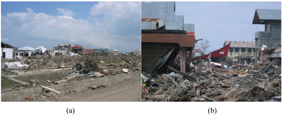
Figure 2.31 Destruction of residential community of timber structures in Banda Aceh, Indonesia (Saatcioglu et al., 2006)
