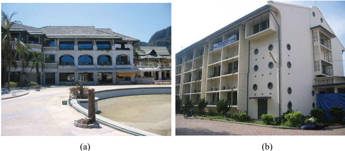
Figure 2.7 Engineered concrete buildings that survived the 2004 Indian Ocean Tsunami without structural damage (Saatcioglu et al. 2009): a ) hotel on Phi-Phi Island, Thailand; and b ) Banda Aceh, Indonesia.
