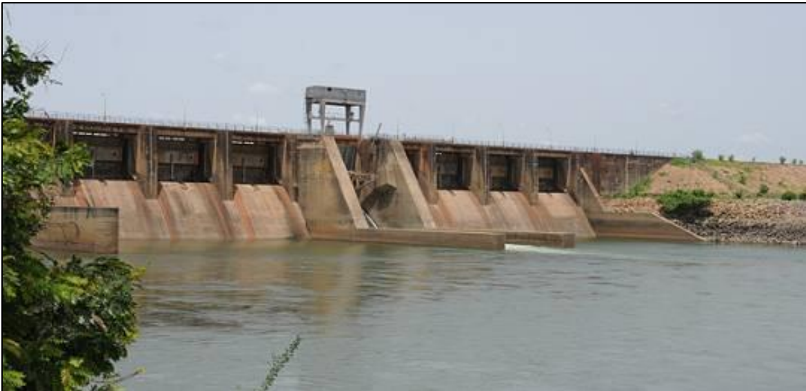
Figure 10: Sélingué Dam. Reprinted from: https://www.iied.org/files/styles/main-image/public/dam_Lucile_web_0.jpg?itok=f8RTAIQh .
