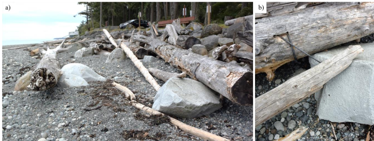
Figure 7 – Examples of Large Woody Debris anchored into the foreshore using cable and rock ballast in Comox, BC. (a) View looking alongshore and (b) close-up of the anchoring system.
