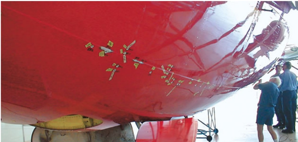
Figure 1: Damage caused by lightning moving along an airplane causing many exit locations [2].
