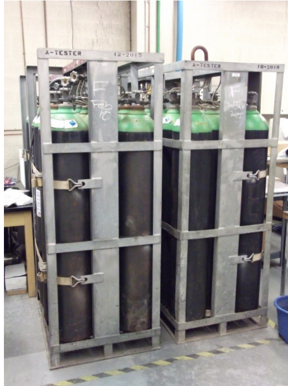
Figure 83: Nitrogen bottle reservoir (bottle pack).
