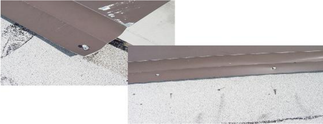
Figure 1.3 Pull-out of the nail and deformation around the nail area (reproduced from Baskaran 2011)
