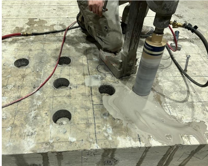
Figure 2.1: Extracting concrete cores
