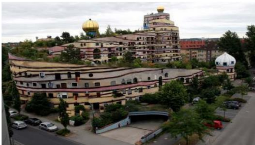
Figure 1-1: Waldspirale Residential Complex, Darmstadt, Germany [12]
