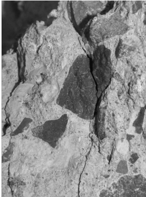
Figure 3-7: Crushed RCA Cylinder showing cracks within RCA
