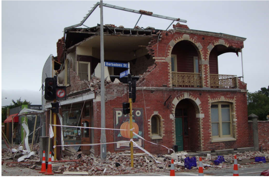
Figure 1-2: Damage to URM after the 2011 Christchurch earthquake, from Wikimedia Foundation by Schwede66 (2011)
