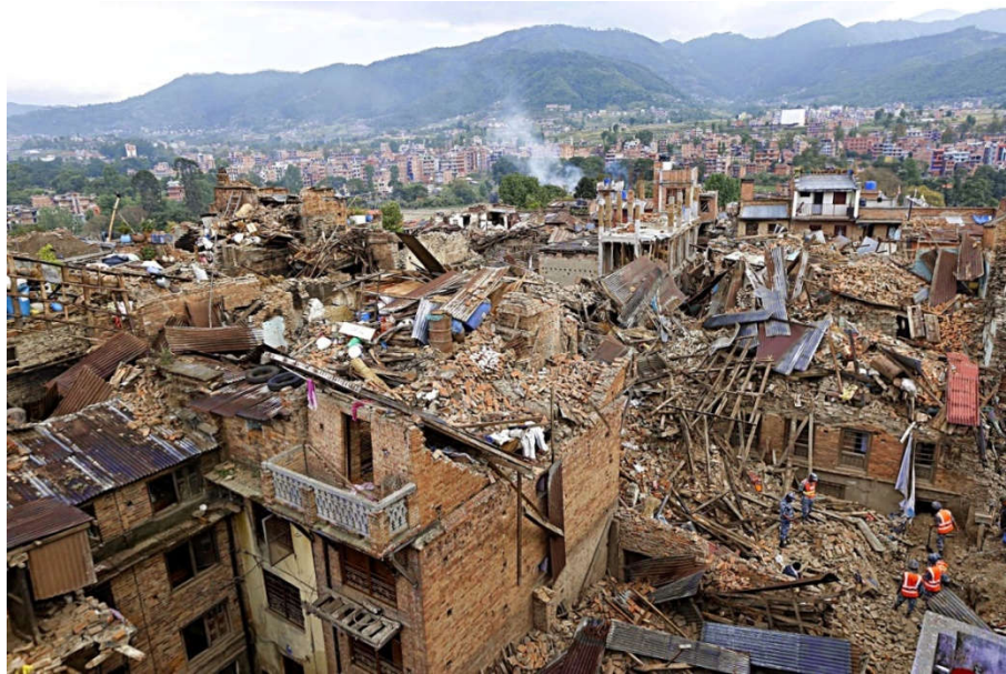
Figure 1-1: Damage to URM after the 2015 Gorkha earthquake, from A. Abdullah (2015)
