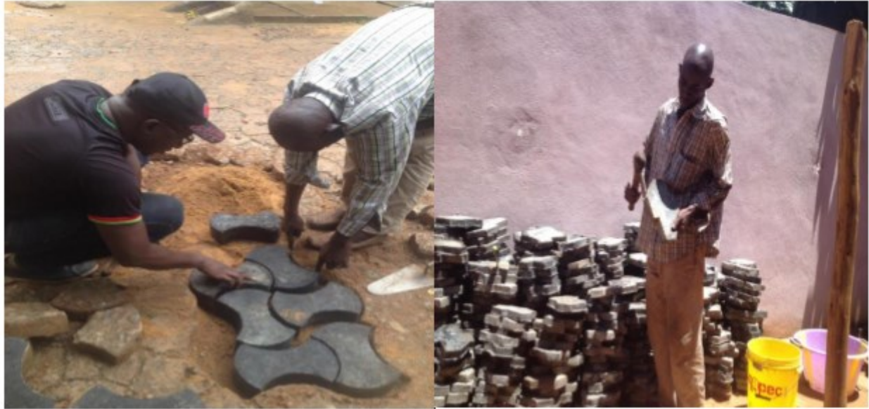
Figure 6-11: Large-scale realizations inside the National Engineering School of Mali using the PWC from our research (Bamako, Mali).
