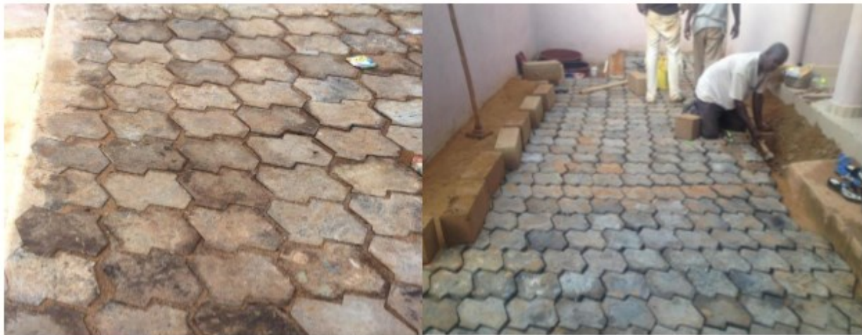
Figure 6-6: Large-scale application of MPB pavers for a) sidewalk and b) house yard rehabilitation in Mali.
