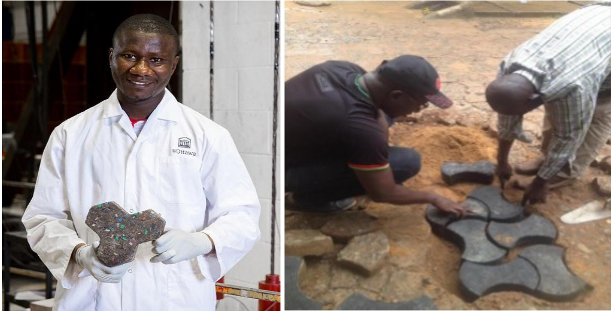
A 3-6: Large-scale construction of PWC in the courtyard of the national engineering school (ENI-ABT) of Mali, with paving stones supporting heavy loads
