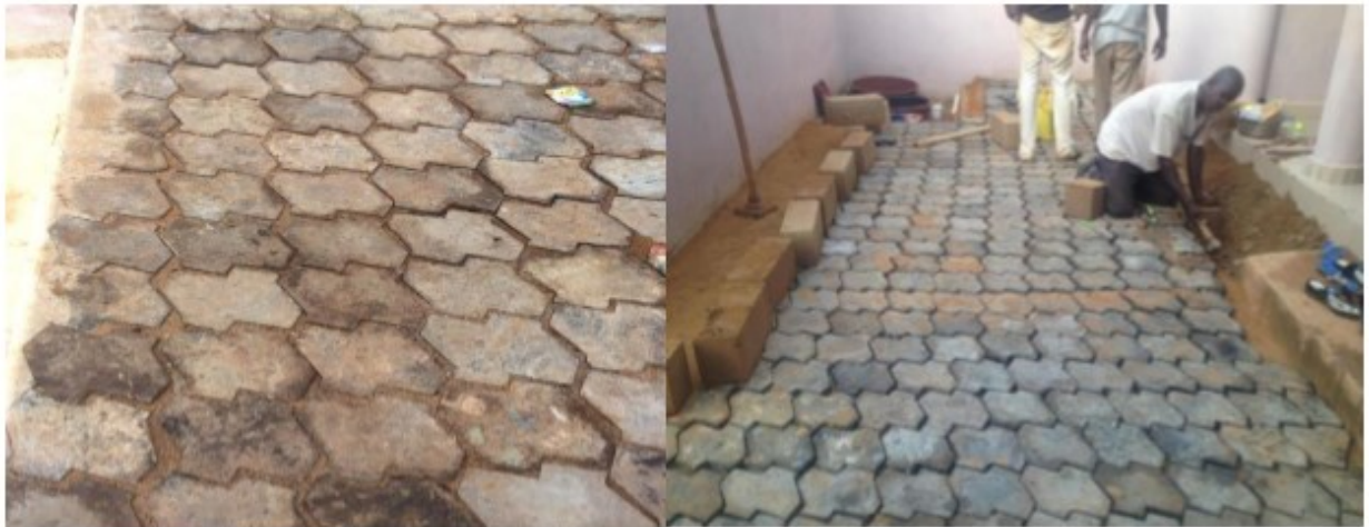
A 3-5: MBP pavers for house courtyard supporting light loads in Bamako.
