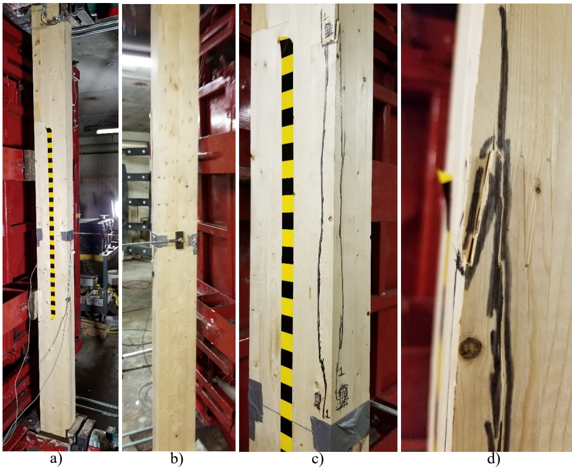
Figure A.12: a) Specimen before test GL2.1 b) Undamaged right side, after test c) Cracking and minor laminate failure d) Detail image of finger-joint failure
