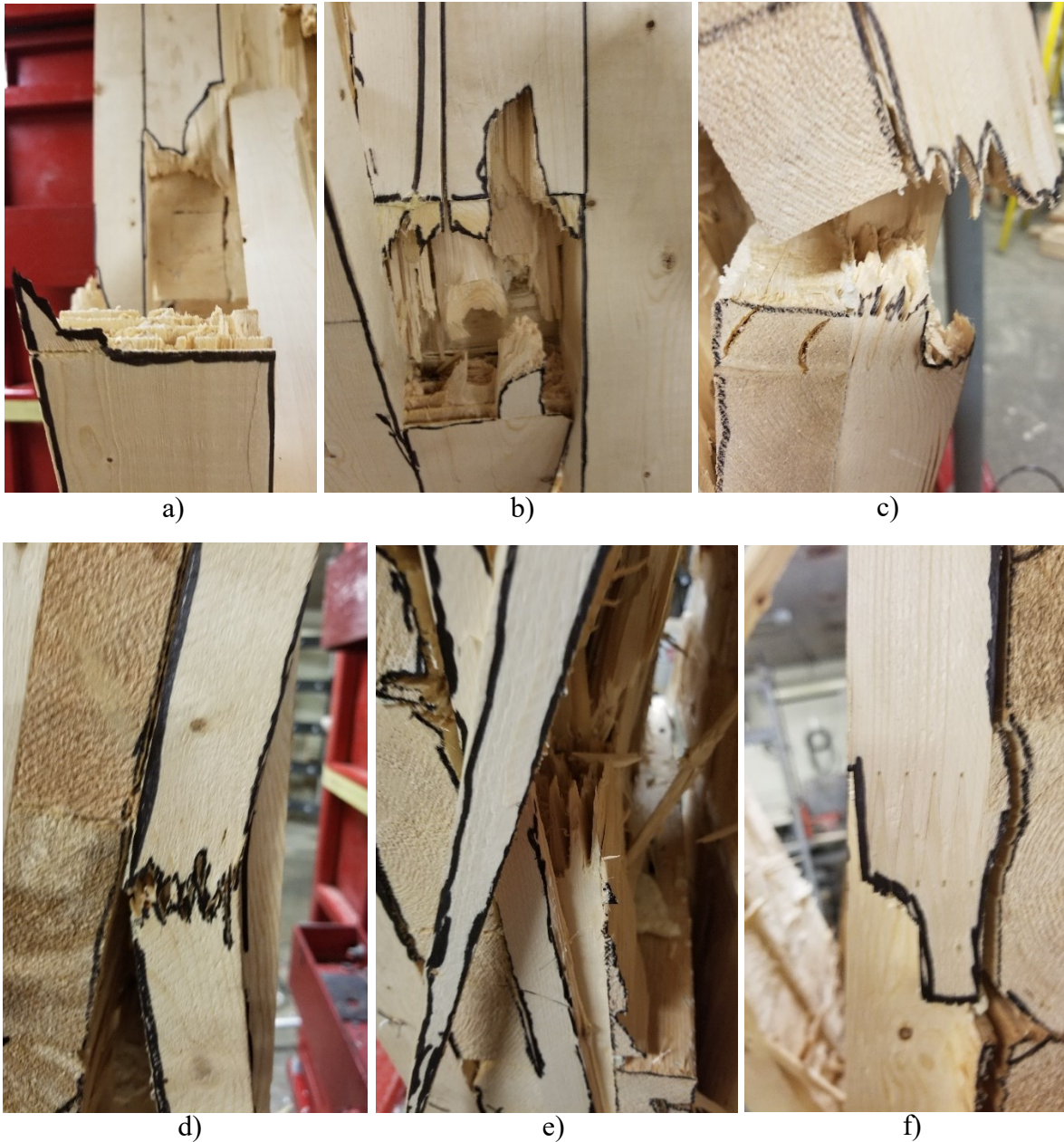
Figure A.44: CLT1.1 Finger joint failures: a) Left tension face b) Lower tension face c) Left side, fifth ply d) Right side, first ply e) Inner lamination f) Right side, fifth ply
