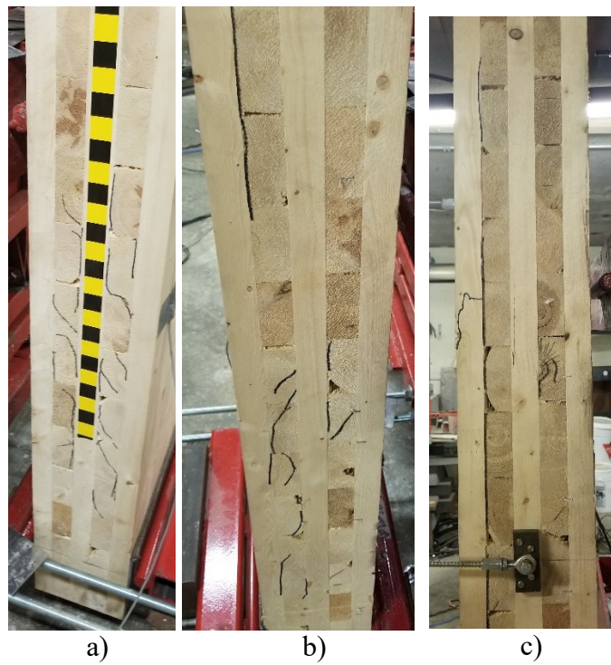
Figure A.55: Transverse cracking details for shot CLT2.1: a) Left side, bottom b) Right side, bottom c) Right side, top
