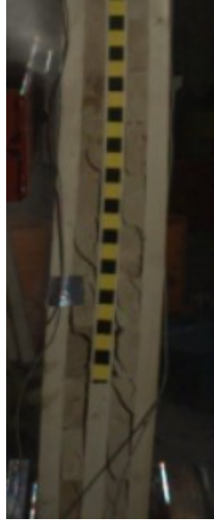
Figure A.56: Formation of rolling shear cracks during test CLT2.1, 24 ms
