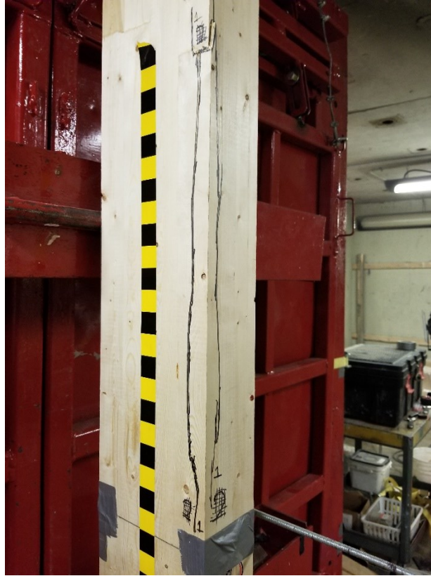
Figure 4.4: Minor splitting failure in test GL2.1, post-test
