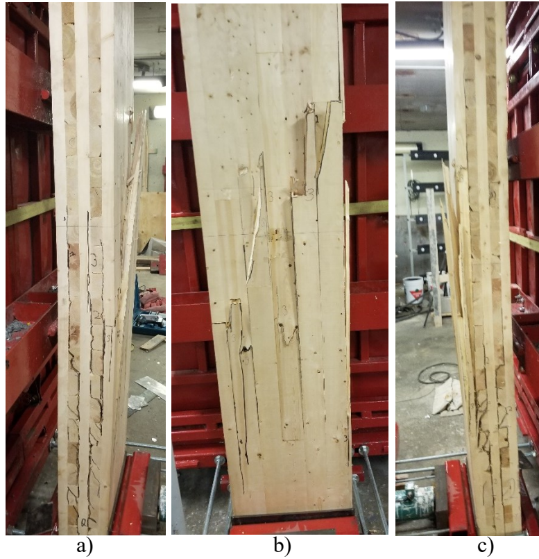
Figure A.68: Final state of specimen after shot CLT2.3: a) Left side b) Tension face c) Right side
