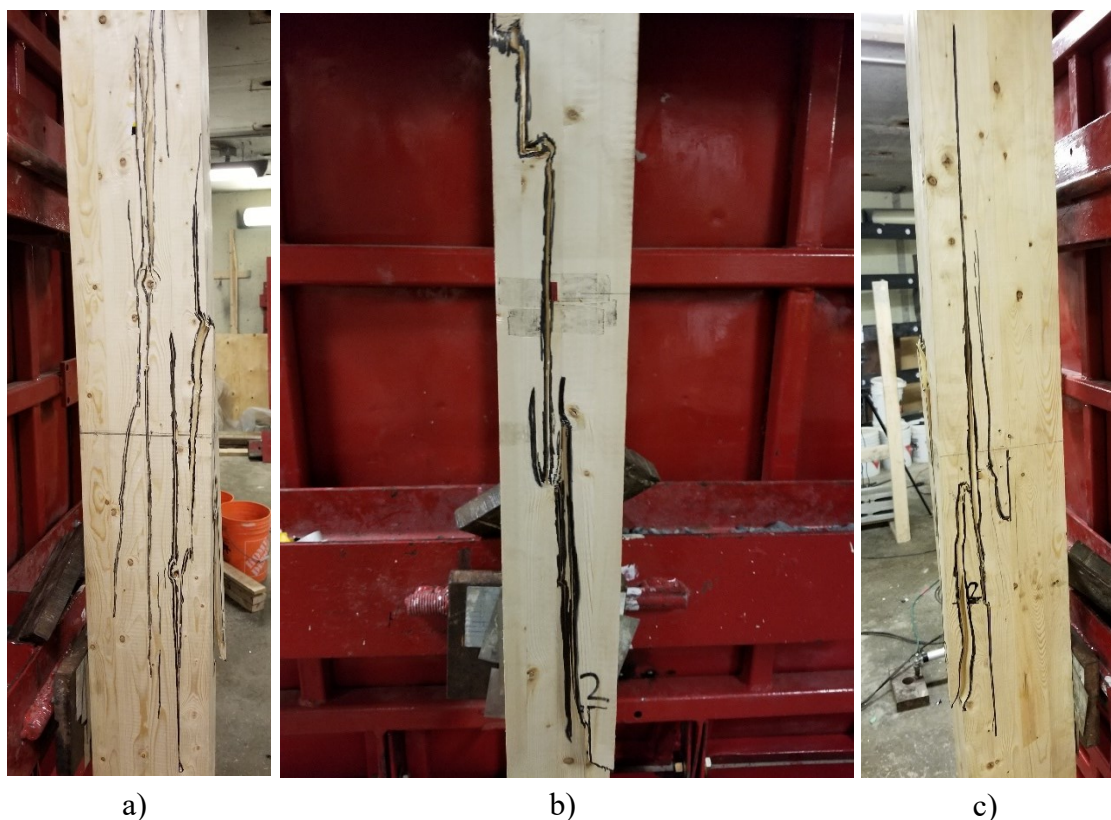
Figure 4.8: Failure cracks for test GL3.3: a) Left side b) Tension face c) Right side
