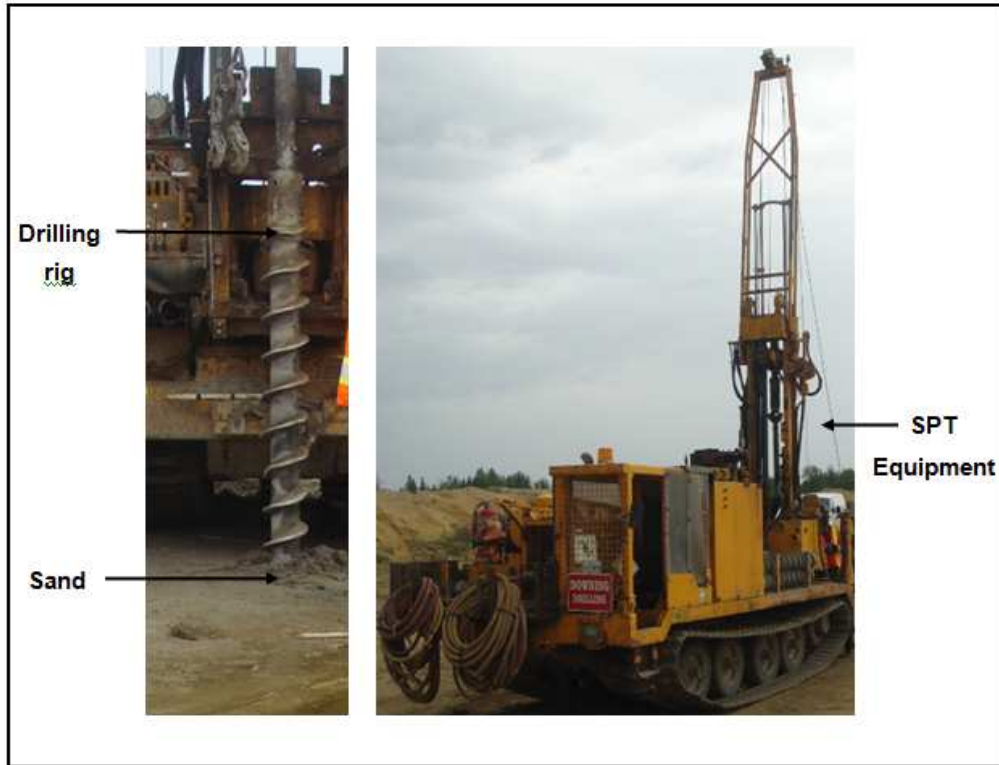
Figure 4.13 SPT falling model truck mounted equipment used in-situ
